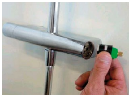
4. Insert the new cartridge
